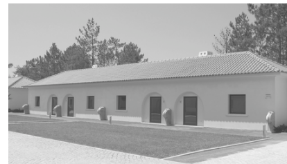
Figure 4: A rehabilitation house at the CMRRC-RP
